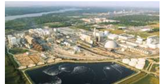
ADM's Illinois Industrial CCS Project: the first large-scale BECCS project
